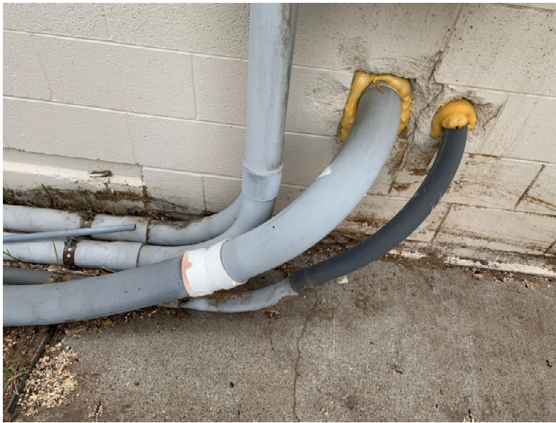
E4: Conduit entrance at dust collector. Shows change in materials at fittings, conduit runs and sealant used.
