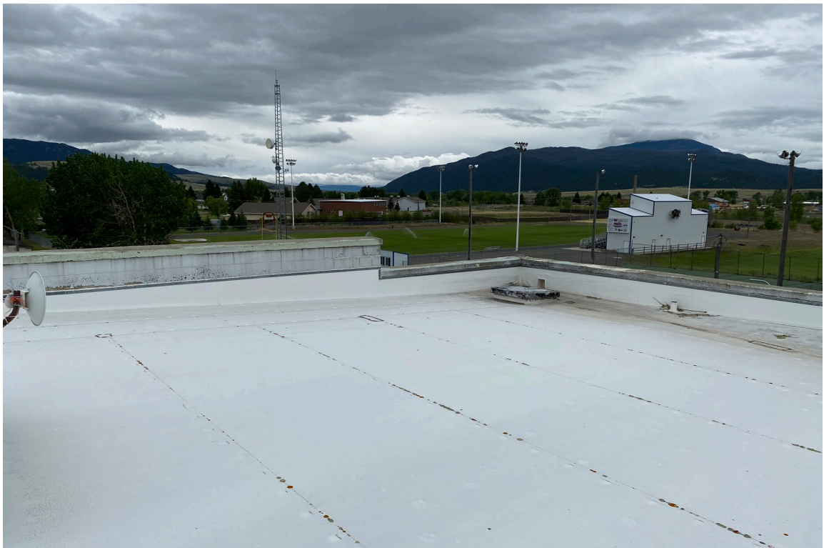
The majority of the existing roofs appeared to be in good condition. This roof, over the Existing (South) Gym, had very little damage and transitions and termination bars were in good working order.
