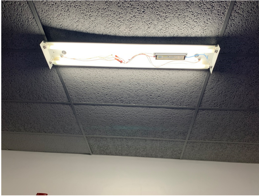
E12: Light in Locker room missing lens
