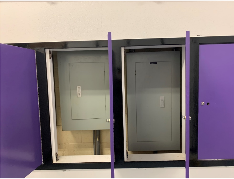
E14: Panels off of Gym lobby enclosed in cabinets. Working space clearances not met.
