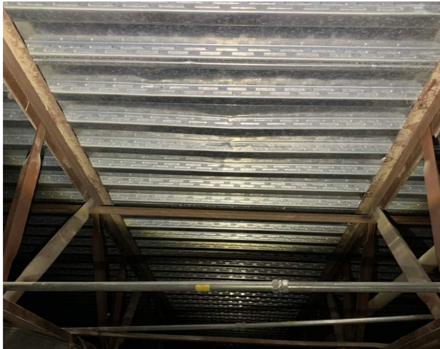
Figure 6. Deformed Metal Deck Below Weight Room (1985 Addition)
