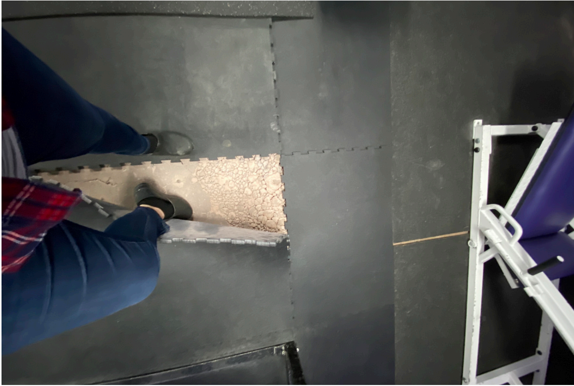
Crumbling composite concrete deck of weight room. Heavy plates and dropping of weights has resulted in severe deterioration of the deck. While this is not a structural problem, it is recommended that the weight room be moved to a floor with a thicker concrete slab.
