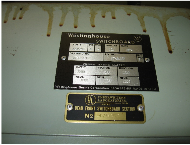
E1: Main Distribution Board showing liquid substance leaking from/onto equipment.
