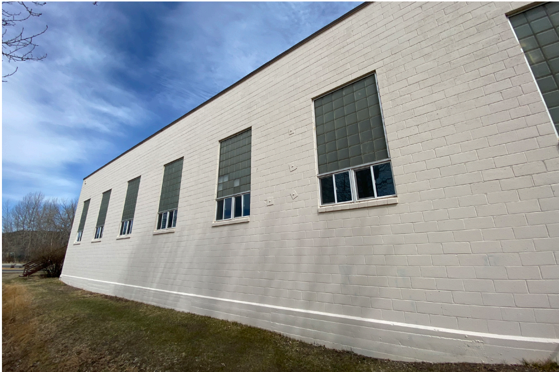
South side of Existing Gym, next to irrigation canal from the Boulder River. Masonry block is holding up well, and paint appears new.
