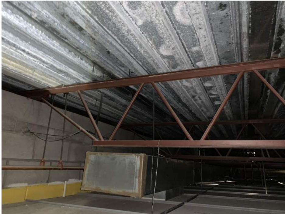
Figure 3. Roof Framing Above Wrestling Room (1985 Addition)
