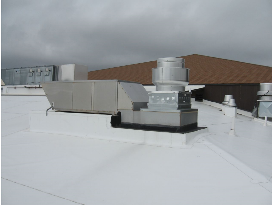
M11: Kitchen Makeup Air and Exhaust Fan
