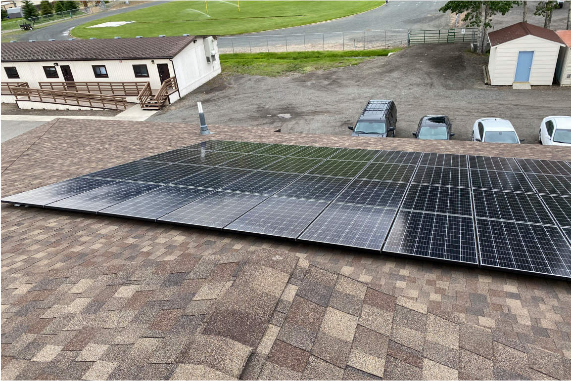
South Library roof, looking towards modulators and storage sheds. Shingles on the Library roof appeared in good condition. Modular roofs had shingles damaged and torn off, mostly from high winds over the previous weekend. Solar panels did not appear damaged.
