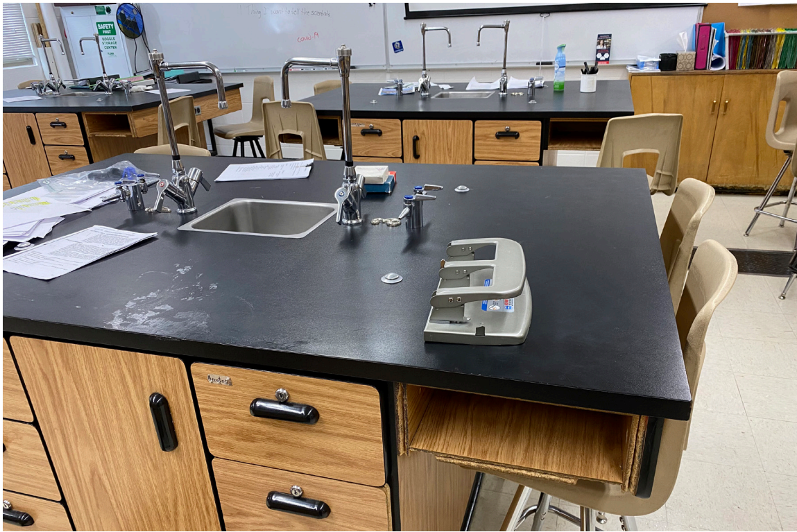
Casework and countertops in the Life Sciences room. While most of these are in good condition, there are areas of wear. This room is too small for a typical science room.
