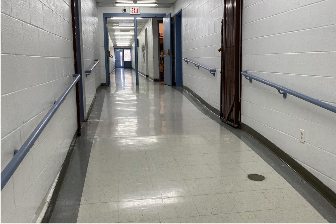
Ramps in main hallway running east-west. Landings, handrails, and slopes all appear to be within current ADA requirements.
