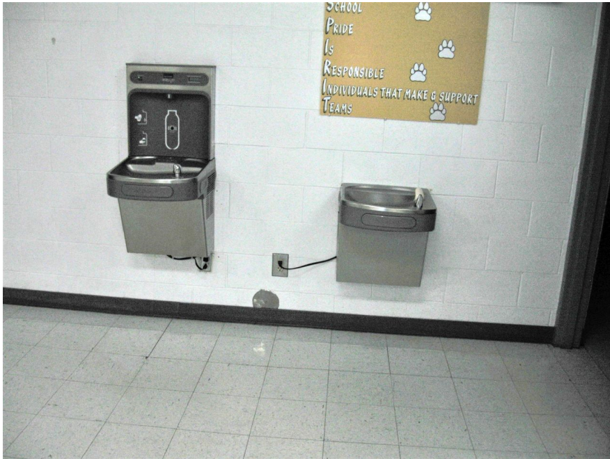
M10: Electric Water Coolers
