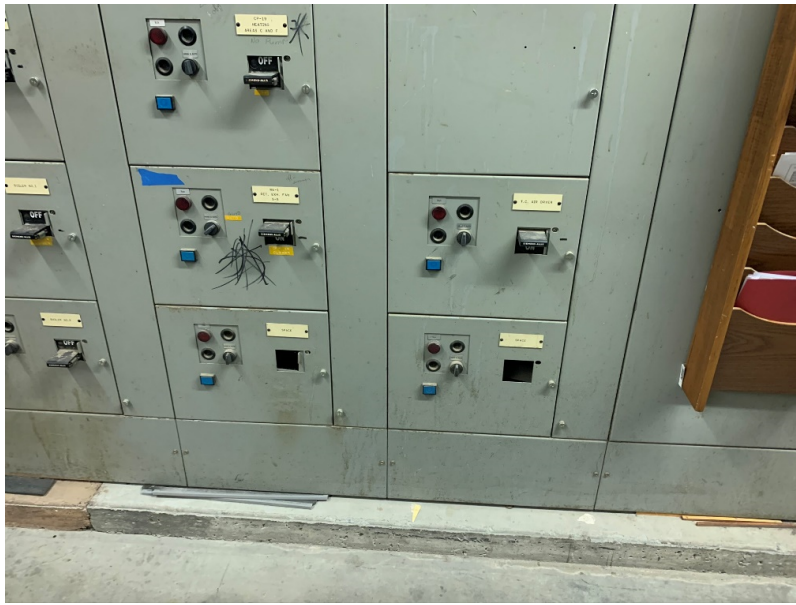
E2: Missing cover plates on MCC buckets need to be repaced.
