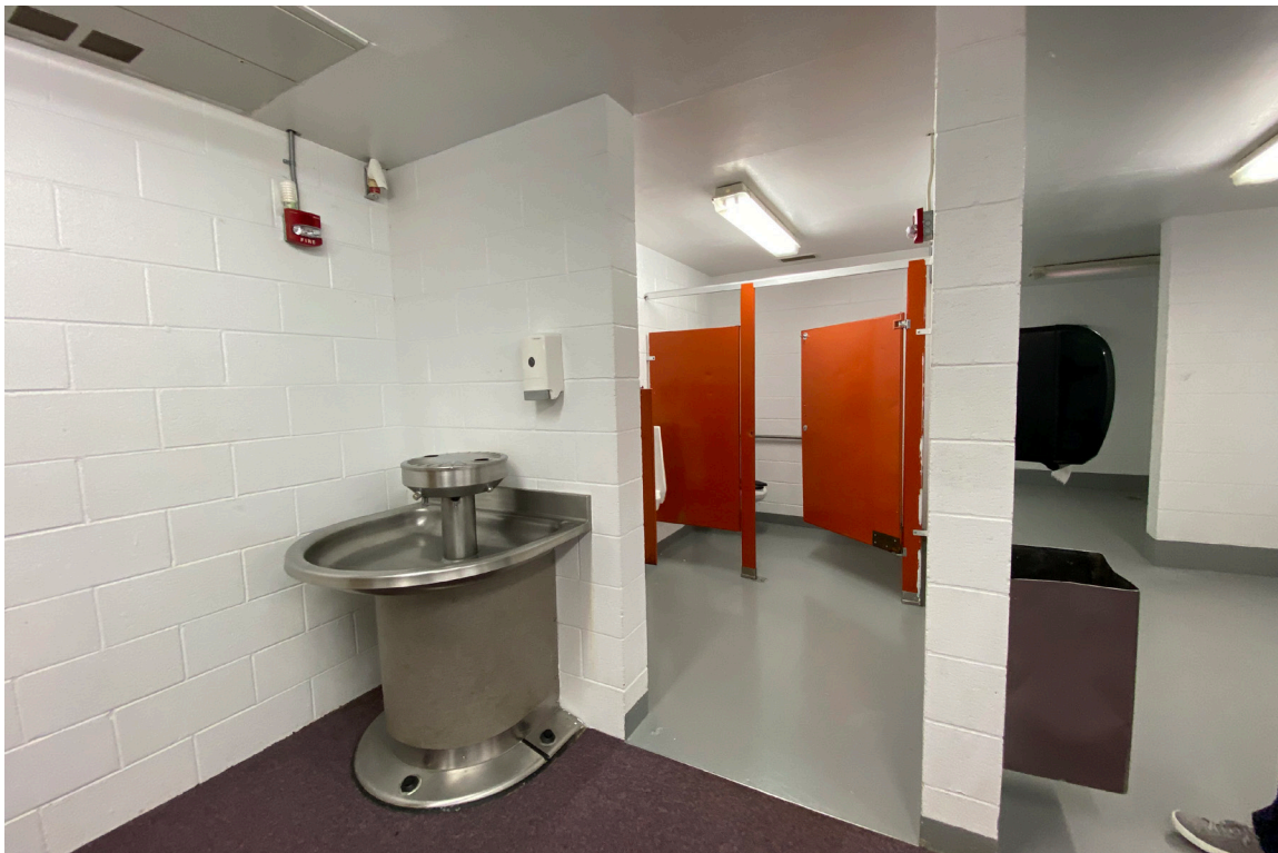
The main floor locker rooms with hand wash station. These stations are designed to serve students around its perimeter, but placement next to the CMU block wall limits access. This reduces the number of required lavatories per the International Building Code (IBC) and amendments per the Administrative Rules of Montana.
