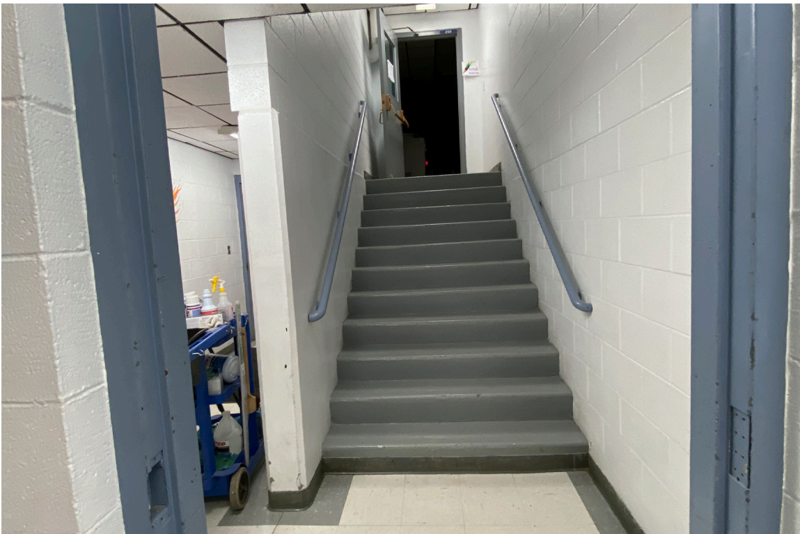
Stairs leading up to the Band Room from the Hallway. There is no accessible route to the Band Room, limiting access to those with mobility issues.
