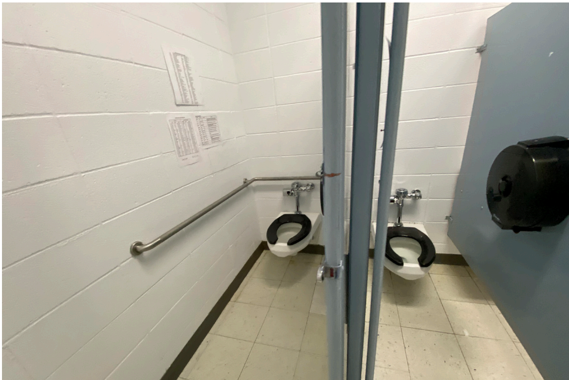
A typical ADA stall in the school. While the grab bars do provide assistance in transferring to the seat, these stalls are not up to current ADA design guidelines.
