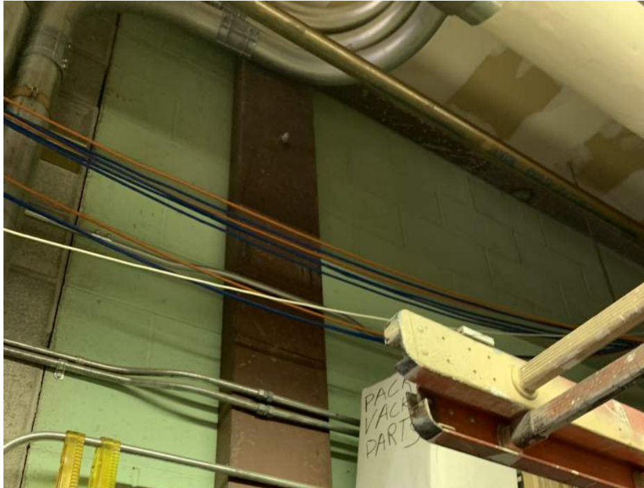
Figure 13. Channel Ledger and Column at Interface Between Mechanical Room and Wood Shop
