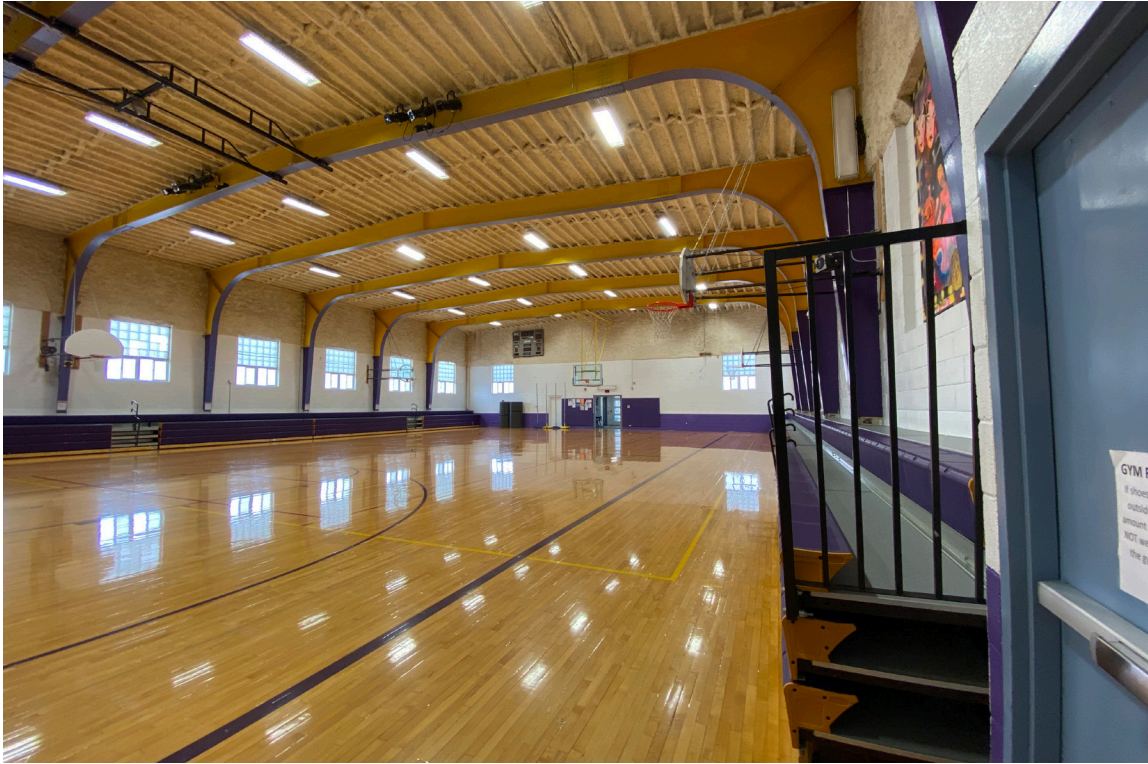
Existing (South) gym. This space is reportedly loud for drama and theater presentations, and is shared with athletics. The spray insulation on the ceiling needs to be verified for flammability and smoke spread, as the design team is not confident it should be left exposed.
