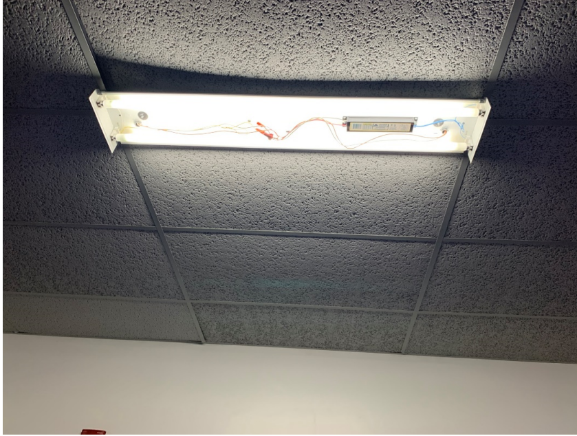
E15: Damaged fixture in weight room.
