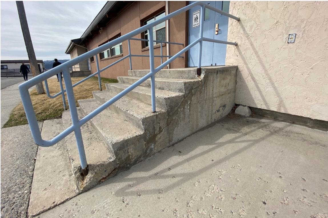
An area of spalling concrete around handrail posts. While not dangerous or against accessibility codes, continued wear will eventually lead to the handrail dislodging from the concrete. This could give way under lateral load when in use and cause injury.
