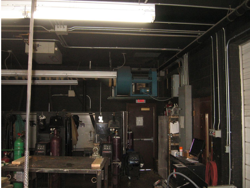
M21: Welding Shop Exhaust Fan
