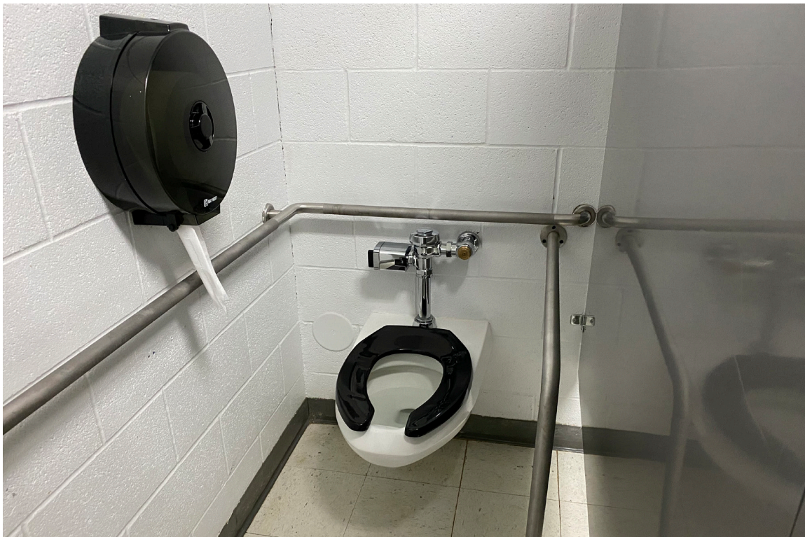
Toilet fixture and stall in restrooms adjacent to Cafeteria seating area. Even though it has several grab bars, this restroom, like most in the school, does not meet current codes for accessibility.
