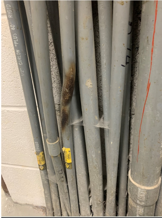
E5: Conduit shows signs of electrical fire and should be investigated by Electrician and replaced.
