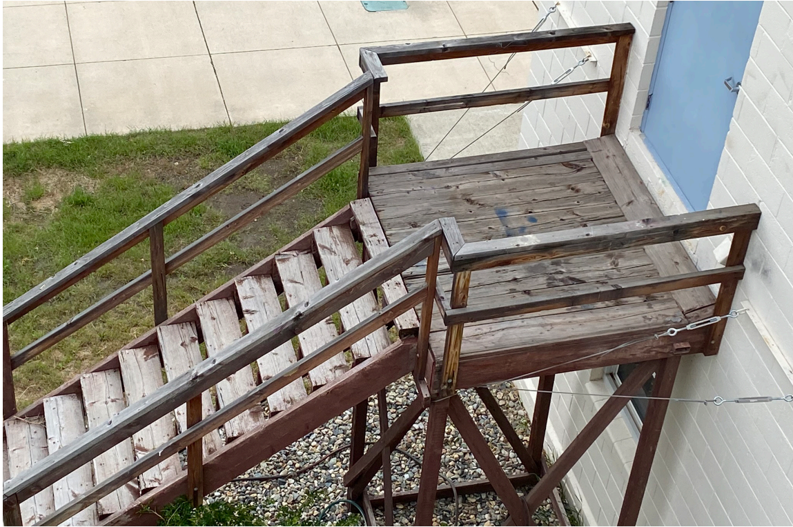
The egress stairs from the Art Room, as seen from the South Gym roof. The wood appears deteriorated and is secured to the building with cables. This stair does not comply with current accessibility codes and needs to be replaced with a more permanent stair.
