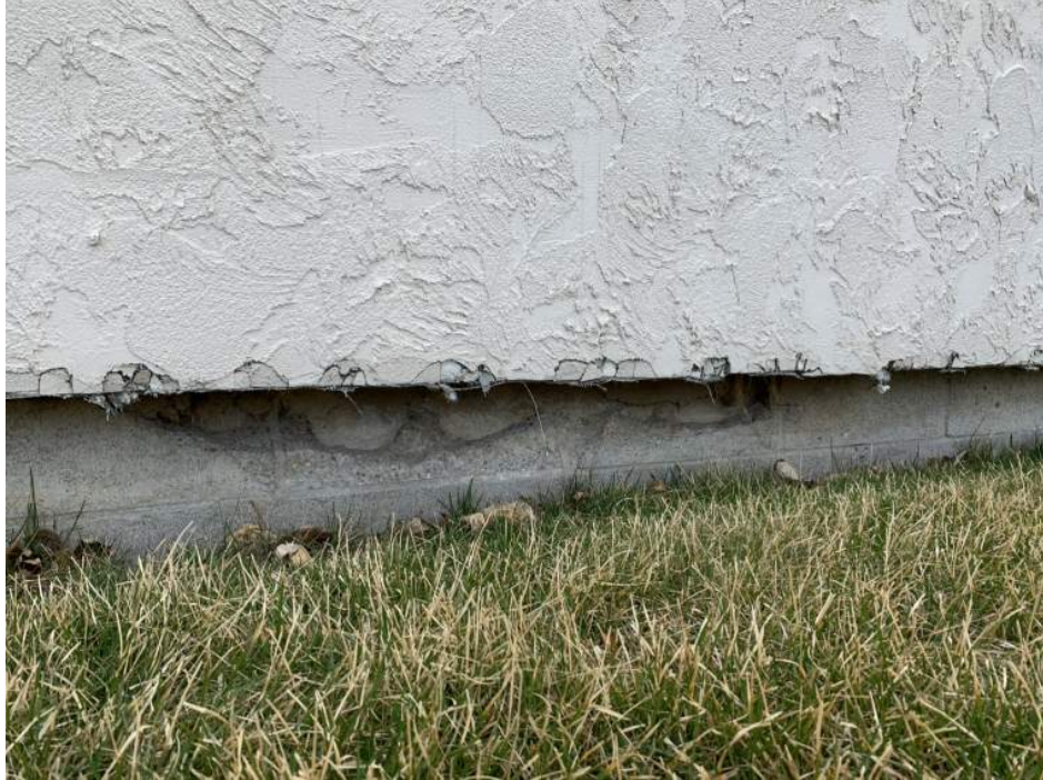
Figure 7. Exterior Foundation Wall Damage at 1985 Gym
