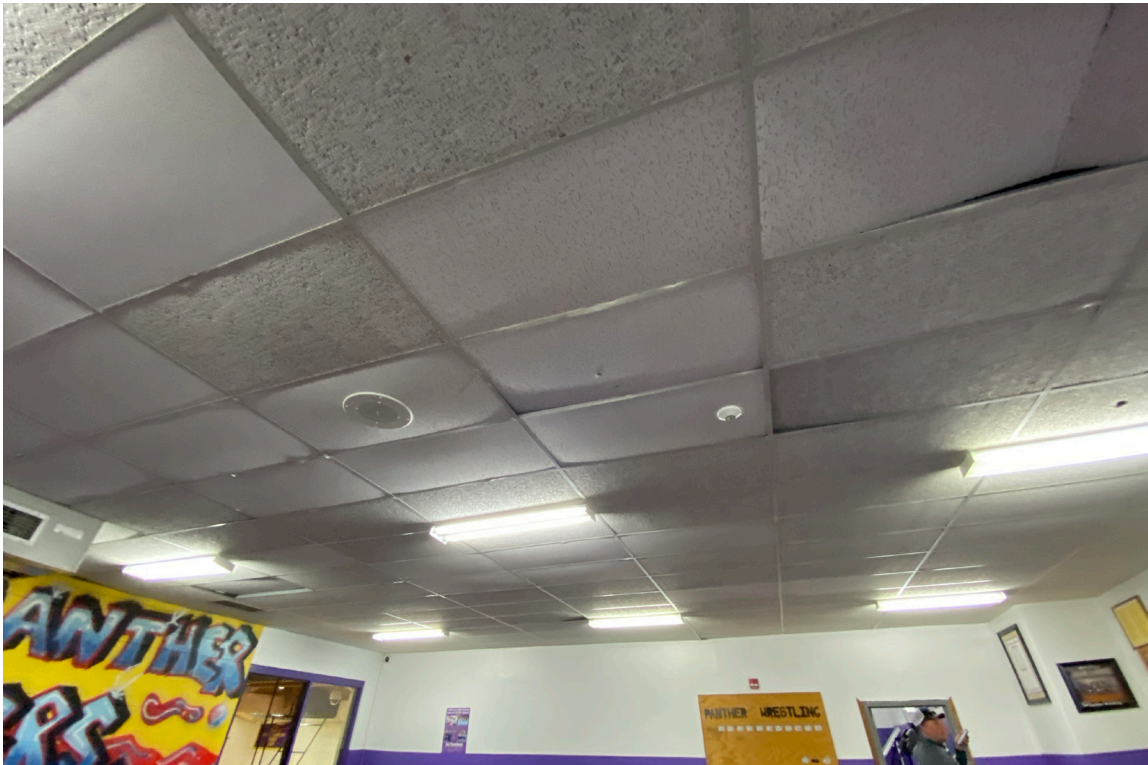
Ceiling tiles in the wrestling room are severely warped and discolored, from previous roof leaks and excessive moisture. Many areas in the school have the same issue and need to have the tiles replaced.
