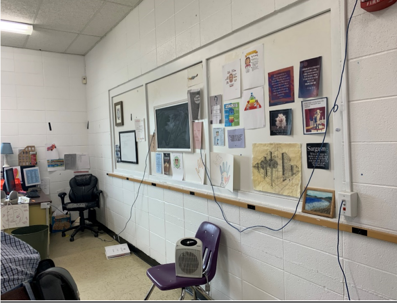
E13: Communication cable draped across teaching wall to desk.
