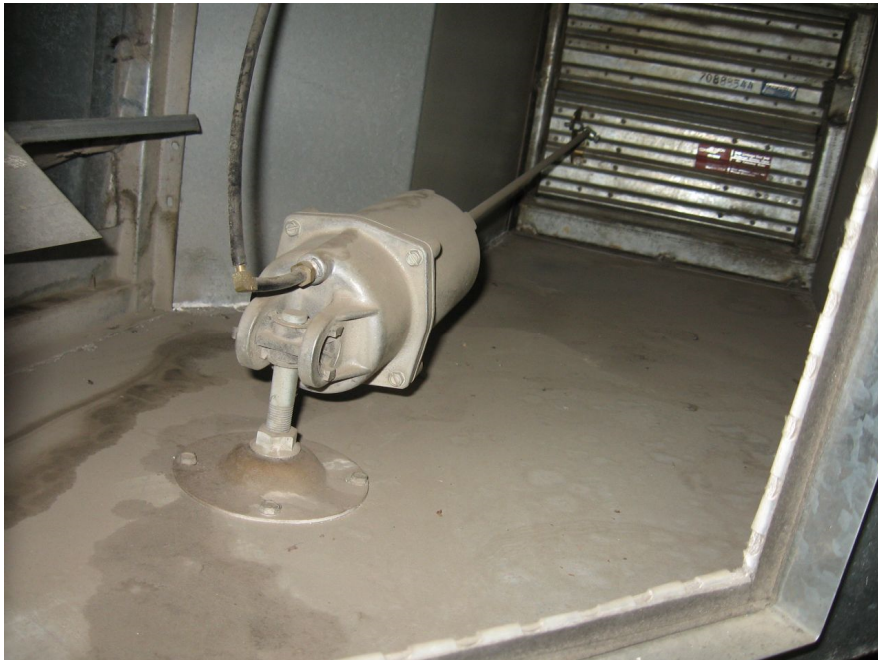
M16: Furnace Outdoor Air Pneumatic Damper
